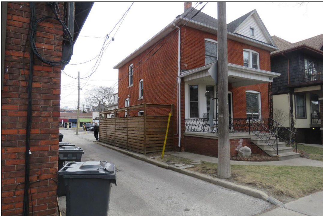
Figure 6 - Looking east towards 642 Windermere Road from Windermere Road
