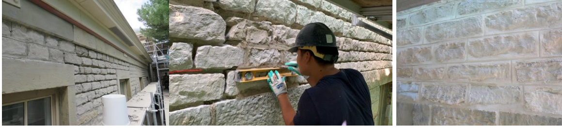
Removal of inappropriate cement mortar for repointing work
