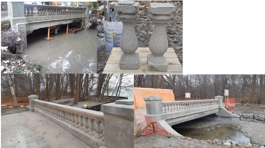
Repair work conducted and the finished work.
