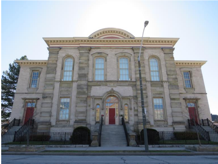
Front view of Mackenzie Hall
